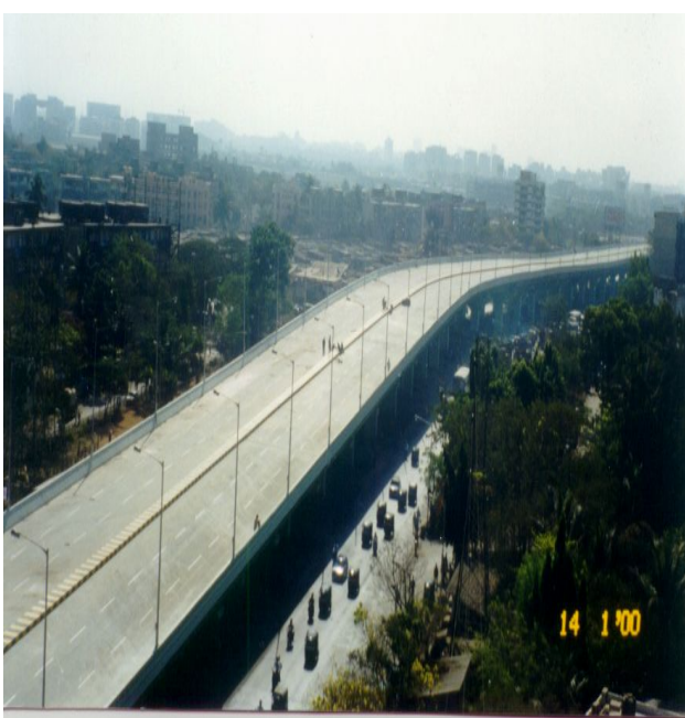
Flyover at Kalina and Vakola Junctions, Bombay, India
