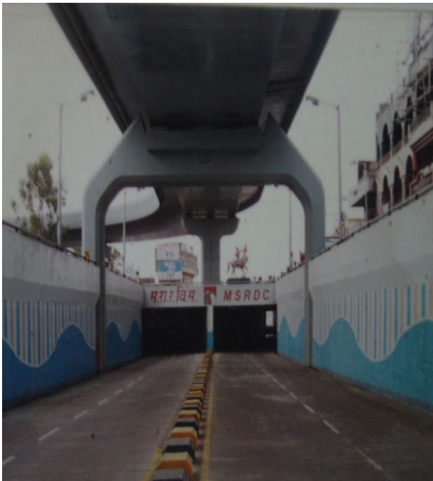
Flyover Cum ROB, Subway and Allied works, Latur India
